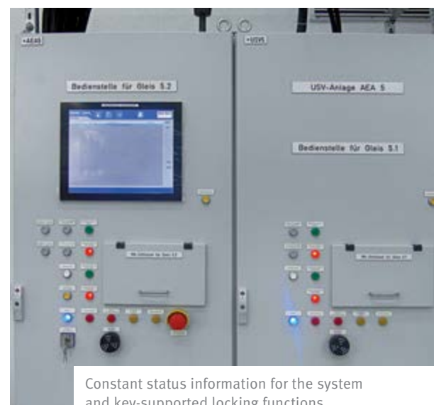
TracFeed® AEA – assures the switch off and earthing of the catenary before work is begun
