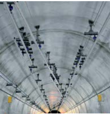
TracFeed® OSS Overhead conductor rail
