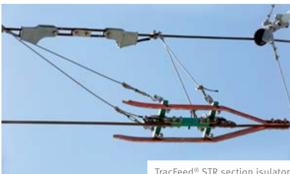
TracFeed® STR section insulator
