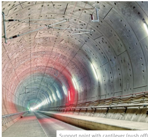
Support point with cantilever (push off)
