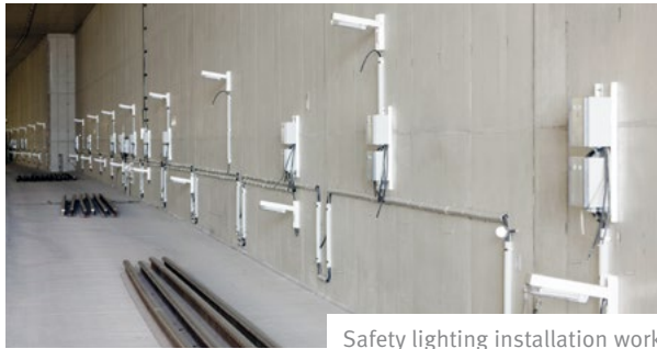
Safety lighting installation work
