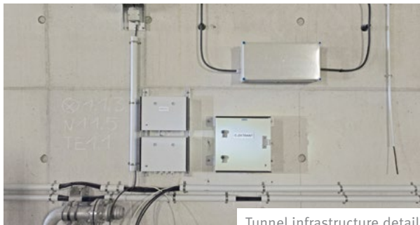
Tunnel infrastructure details
