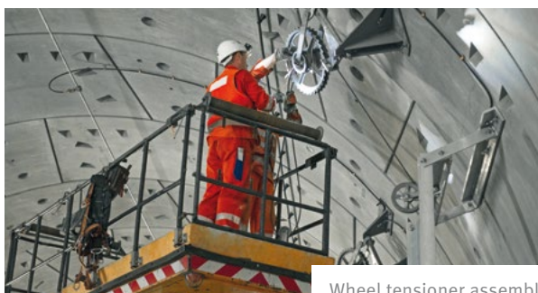
Wheel tensioner assembly
