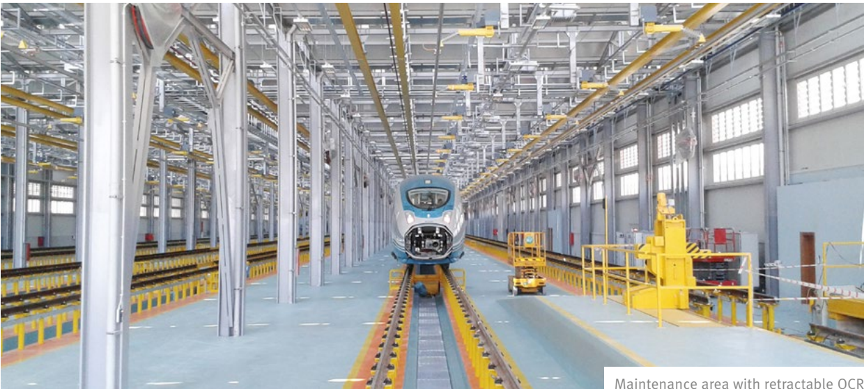
Maintenance area with retractable OCR
